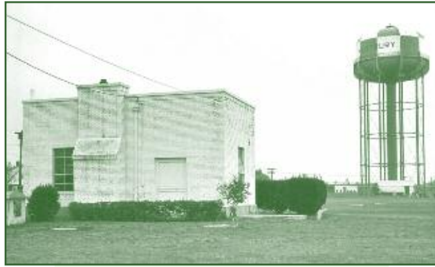
The district's 1-million gallon elevated storage tank, erected in 1947, provides water to the distribution system through the power of gravity. It is slated to undergo a major rehabilitation project in the coming year.
