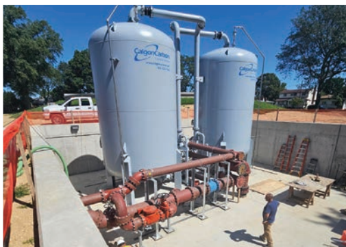
Granular Activated Carbon (GAC) vessels are standing tall at Well 12 & State Street.
